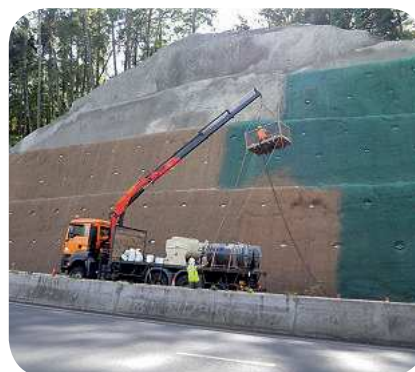
Hydroseeding application (Euro-Tec, France)
